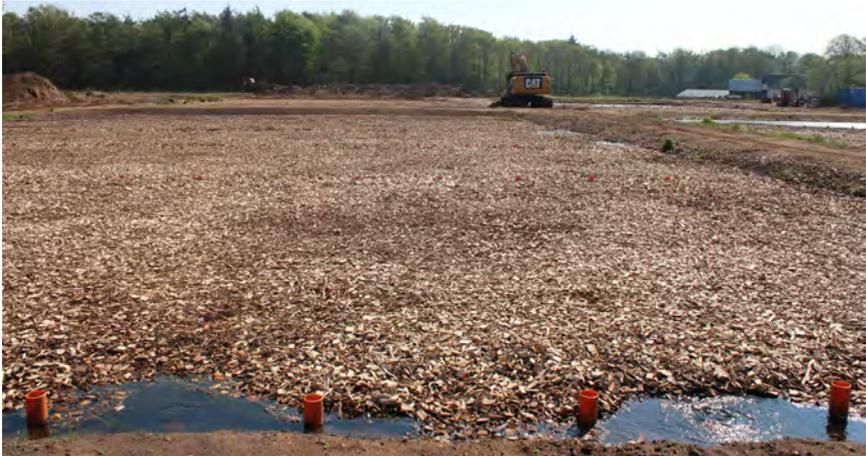
*The filter shown holds 6 000 m<sup>3</sup> woodchip for cleaning 100 L/sec reject water. The woodchip will acts as a carbon source for the denitrifying bacteria transforming nitrate into free nitrogen in an anaerobic environment.*
