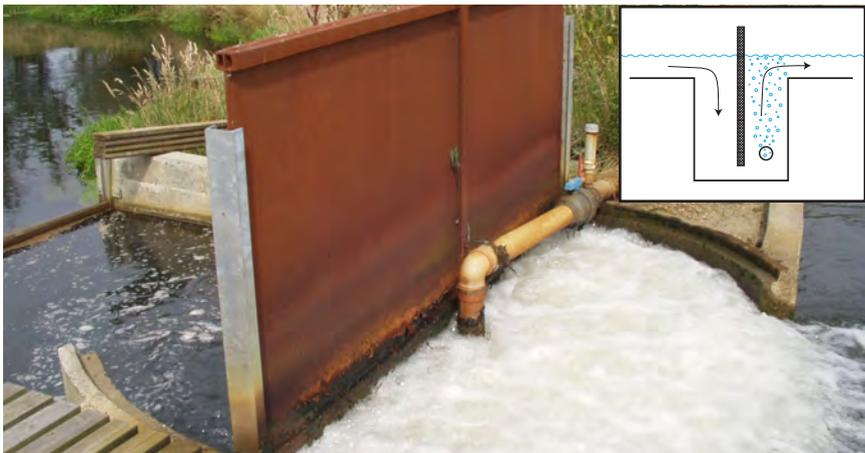
*Air injected at the bottom of the well drags water through the farm. At the same time the water is aerated and degassed.*
