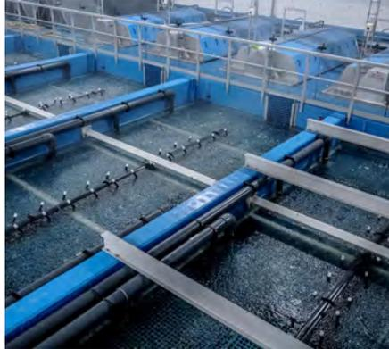
*E.g. the aeration pattern of the fixed bed biofilter shown in the foreground must be stable and uniform.*
